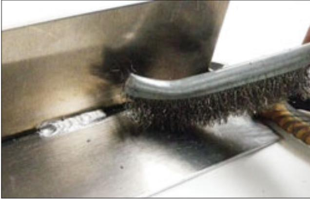
Clean up the weld and remove the carbon from the weld area with a stainless steel wire brush.
