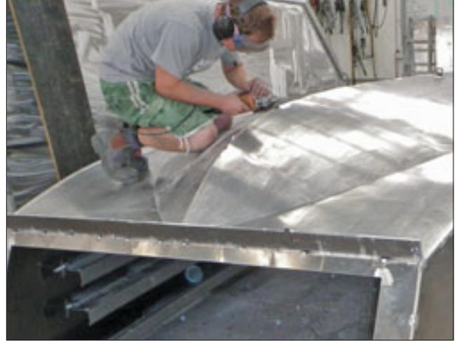
Gareth is preparing the keel weld area by sanding first, then back cutting and cleaning before the final weld.
